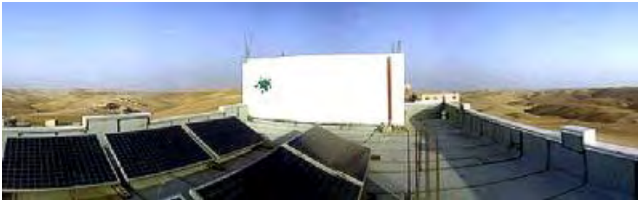
Solar panels on the roof of the Greenstar center in a Bedouin village, on the West Bank.
