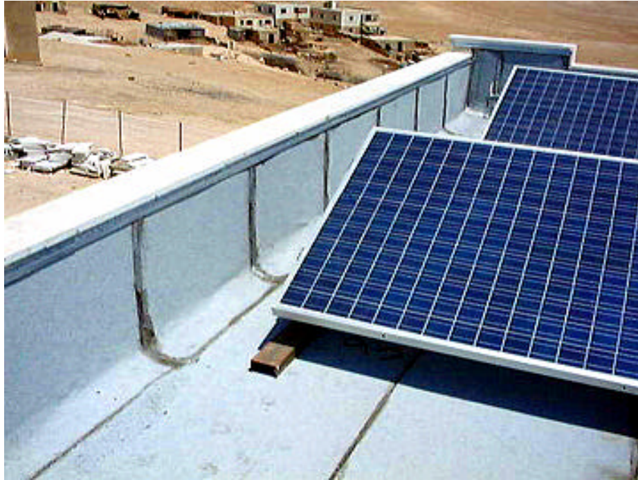
Figure 5: Modules “A” (background) and “E” (foreground) are located too close (i.e. approximately 47 cm) to the western roof parapet (of height 72 cm above roof level). Afternoon shading by the latter will impair array performance. [Further dimensions will be found in Table 6 ]
